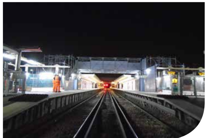
The successful installation of the temporary footbridge in June.
